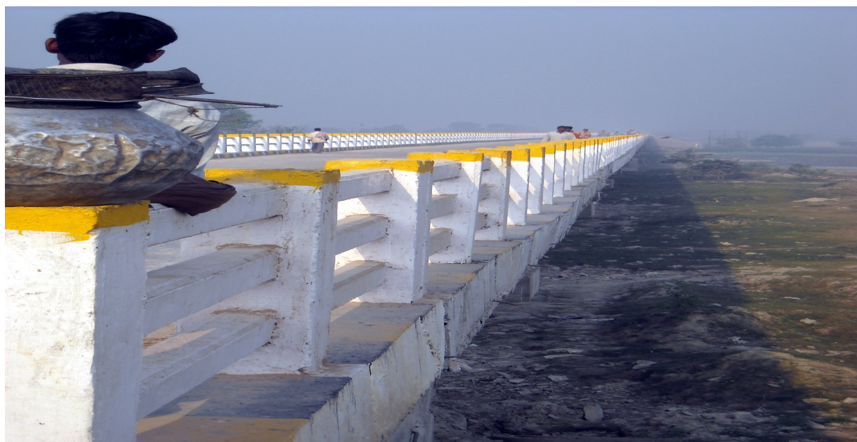
Bagmati River Bridge (Dubba Pool), Sheohar
