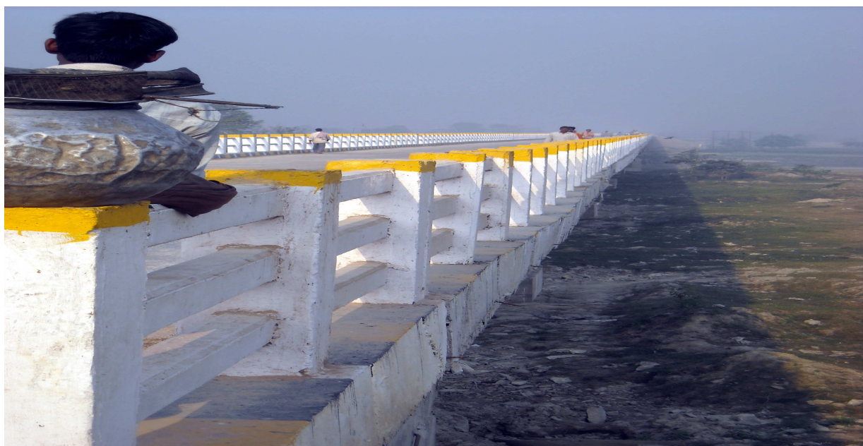
Bagmati River Bridge (Dubba Pool), Sheohar
